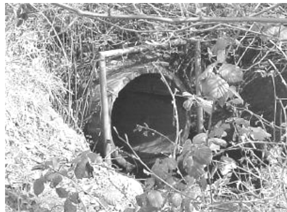
Figure 3. Culvert entrance near the headwaters at the University of Victoria
