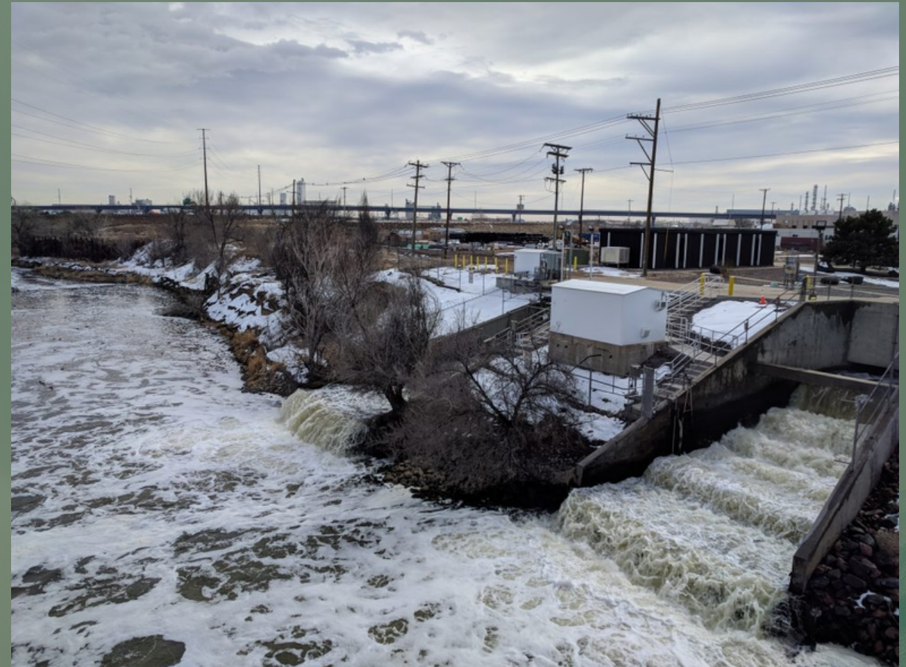
Wastewater effluent into the South Platte River Photo Credit: https://www.watereducationcolorado.org/publications-and-radio/radio/what-not-to-flush/
